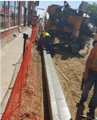
Above: Concrete crews extruding new curb and gutter in front of Home Hardware.
