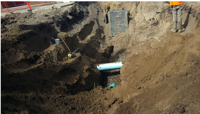
Above: The sanitary main going up the lane passes under the water main to the new sanitary main on 50 Avenue.
