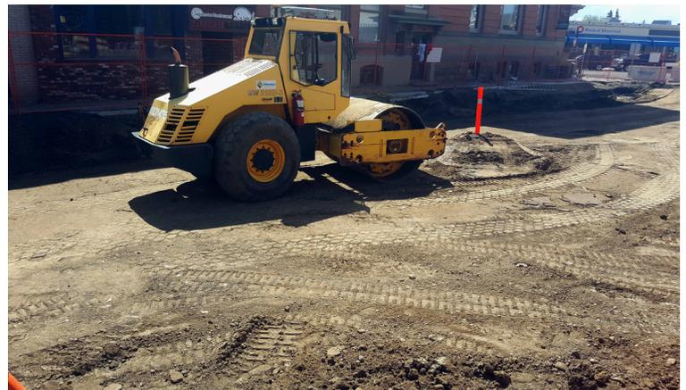
Above: Backfill material is lightly packed to control rainwater on site.
