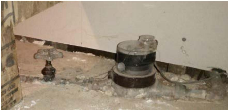
*Figure 1 The water meter and shutoff valves shown encased in concrete.*
